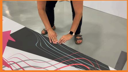
5 To ensure the best fit, go around the perimeter again and smooth any ripples.
