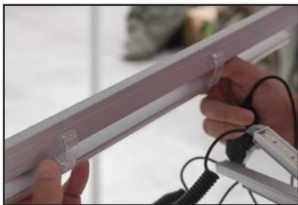
Arrange the black cord connector so it lays flush against the bottom of the center peak pole. Connect each LED light band to desired frame tent scissor piece using the clear connector brackets. LED light bands can attach to frame tent beams in whatever direction you desire (shining up or down).
