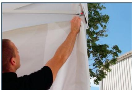
This edge of the wall gets velcroed to the inside of the valance on the roof by starting at one end and attaching it all the way across.
