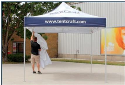
Unfold the wall and locate the top edge that is lined with Velcro. **\*\*Be sure that the wall is being installed into the correct position ie: front, back, sides\*\***
