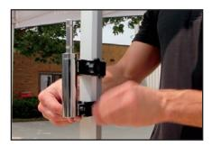
Insert the black knob into the holes in the black bracket and through the spindle. Tighten the knob to attach the spindle to the tent leg. Repeat these three steps with the second black bracket.
