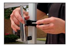
Hold the metal spindle in the opening of the bracket so that the holes in the spindle line up with the hole in the bracket. Install the spindle so that the skinny end is on the top and the wider end is on the bottom.
