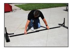
Lay a 4'-A pole and a 4'-B pole end to end between the footplates on the ground.
